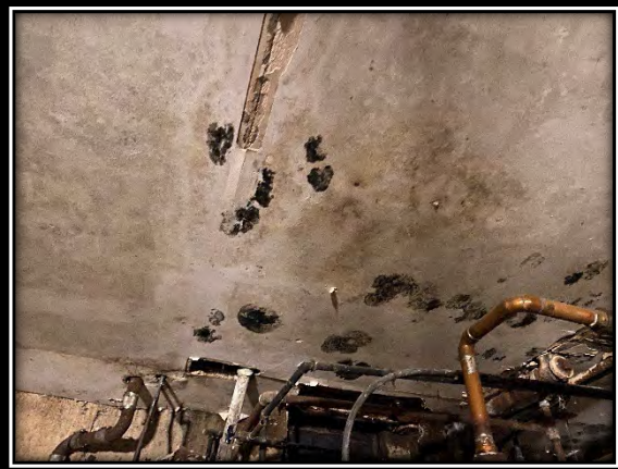
Visible Mold on Ceiling
