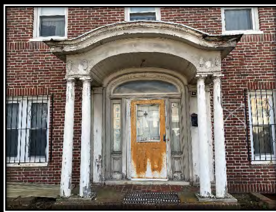
Damaged Front Canopy
