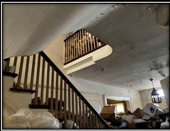
First Floor – Peeling Paint
