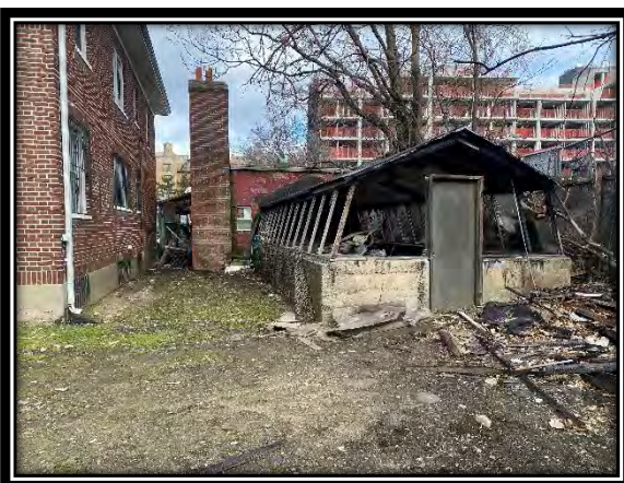
Fire Damaged Storage Shed
