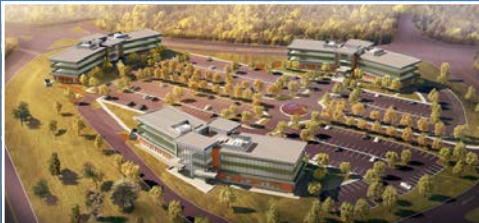
WESTRIDGE CORPORATE PARK 500,000 SF of premier, Class A office space
