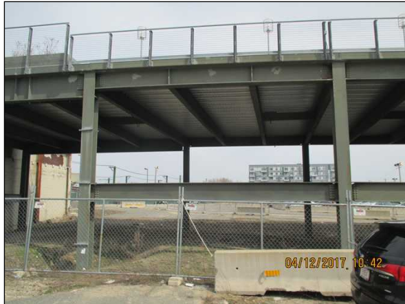
7. Wonderland station footbridge to the north.
