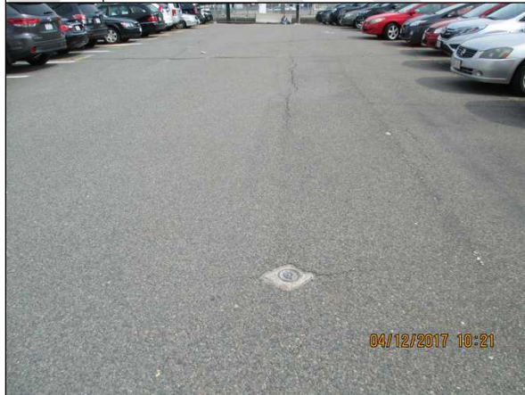
3. Existing monitoring well from West & Sampson's 2010 Phase II ESA
