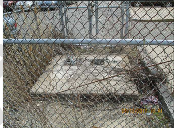
5. Former transformer pad, southwestern portion of Subject Property
