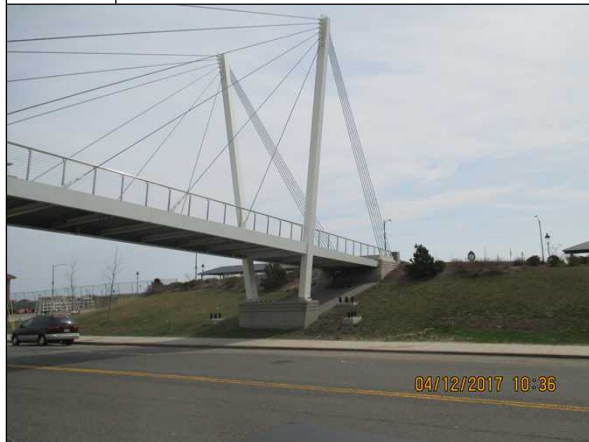
8. Wonderland station footbridge to the northeast and Ocean Avenue.
