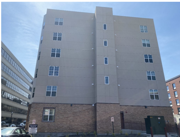
3. View of the north side of the subject property.
