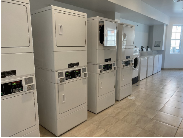
7. View of the resident laundry room.
