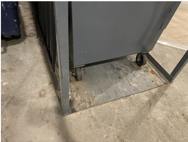
9. View of the trash compactor.
