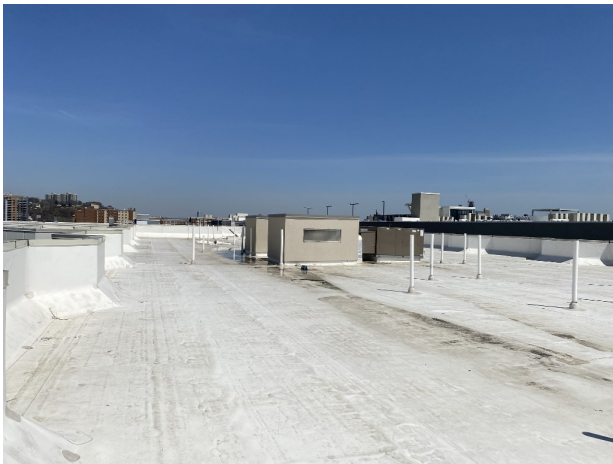
21. View of the roof.
