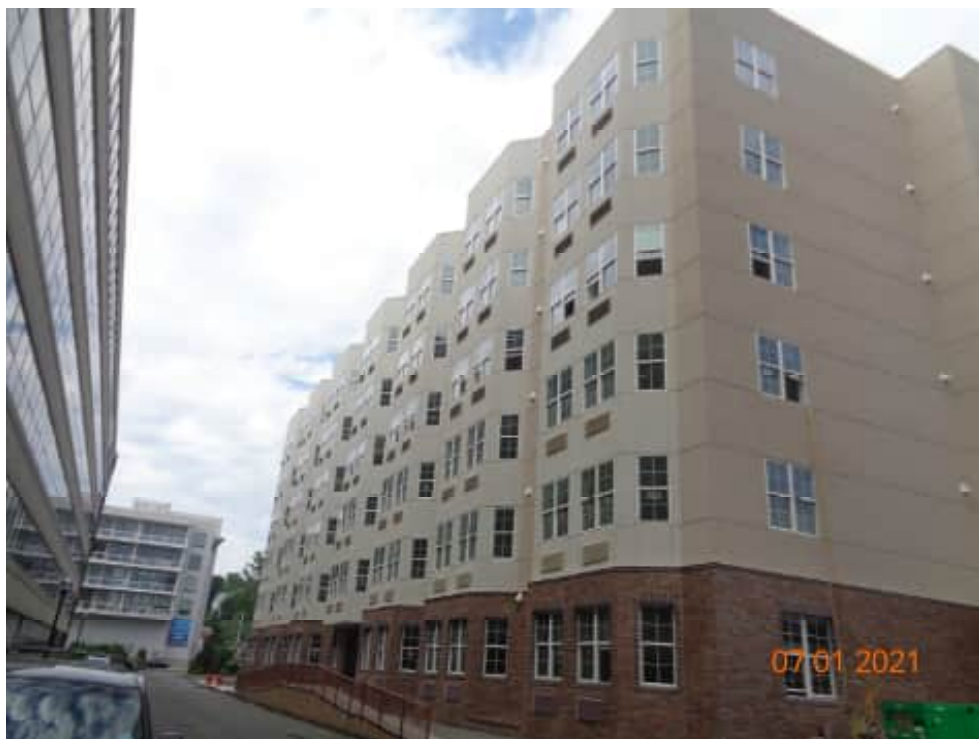
Photo #2 - Rear view of the building
