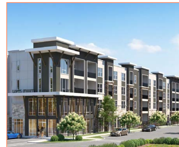
Lofts iThirty - Under Construction 340 Units | Garland, TX
