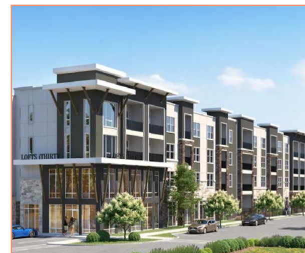
Lofts iThirty - Under Construction 340 Units | Garland, TX
