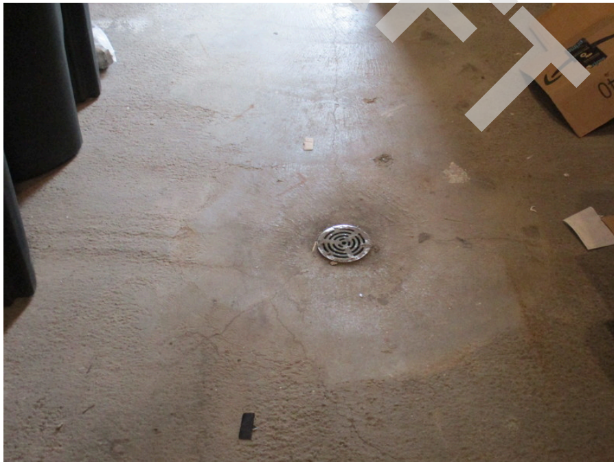
26. Floor Drain in compactor room
