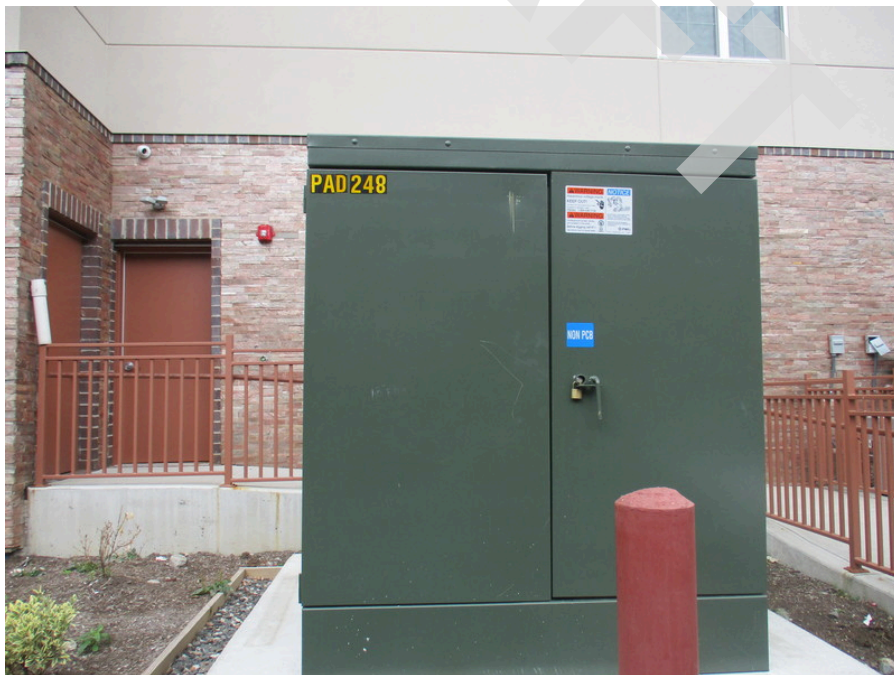
8. Pad-mounted transformer
