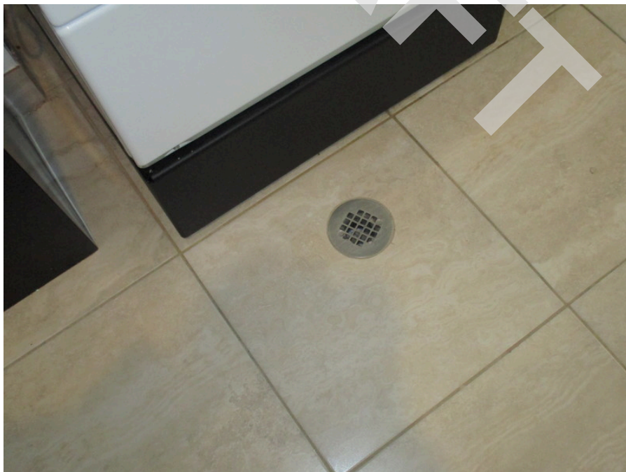
22. Floor Drain in Laundry Room
