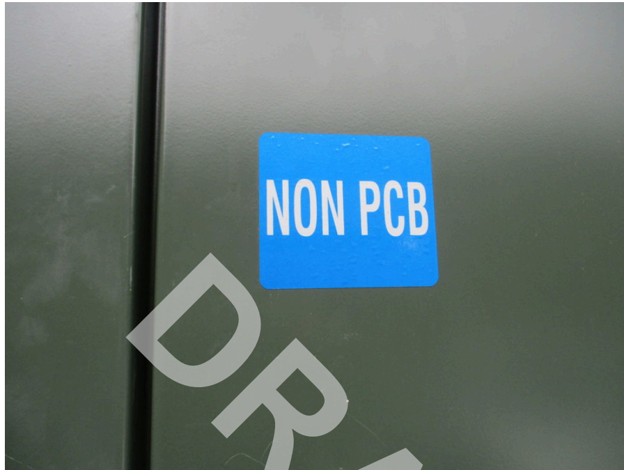
9. Non-PCB label on transformer.
