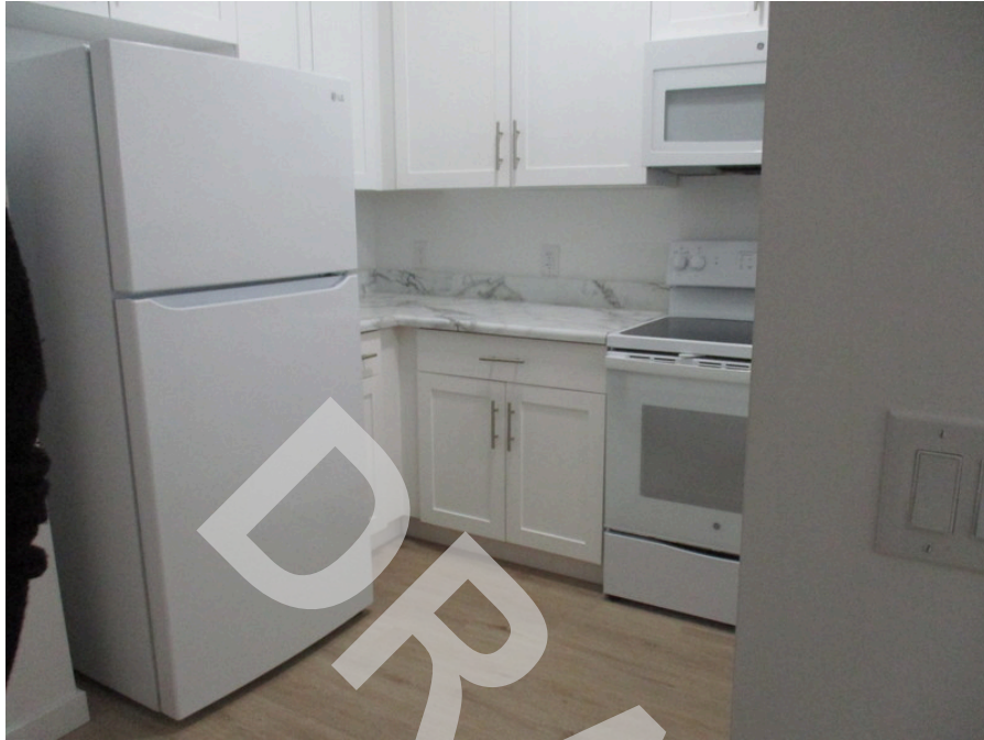
39. Vacant unit kitchen
