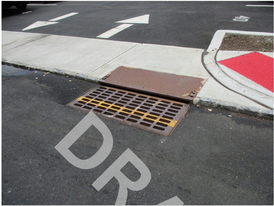
5. Typical curbside stormwater drain
