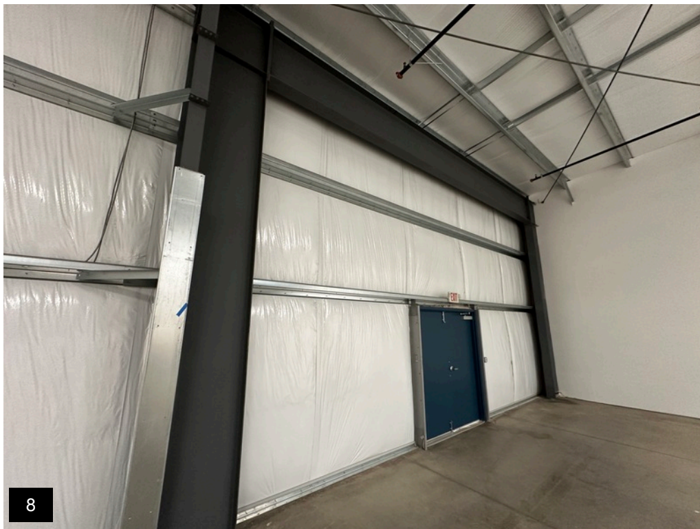
The typical longitudinal steel moment frame.
