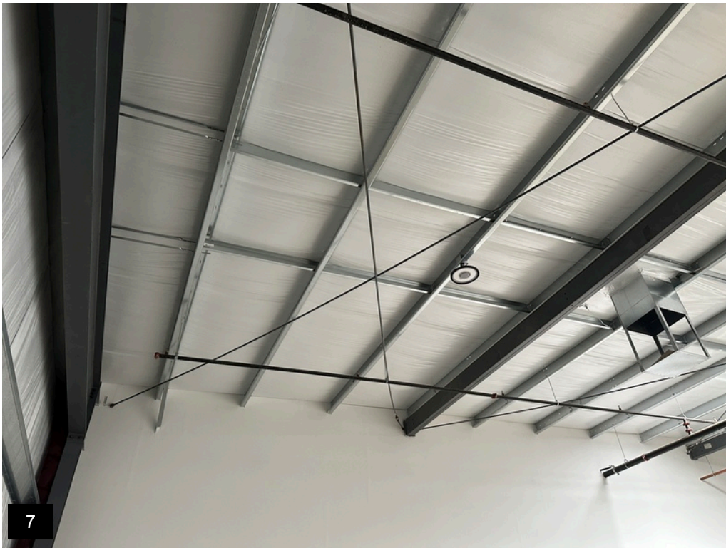
The typical roof tension-only cable diaphragm bracing.
