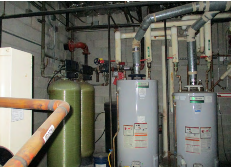
Photo 17 - View of water heaters and water softeners in the surgical center building mechanical room.
