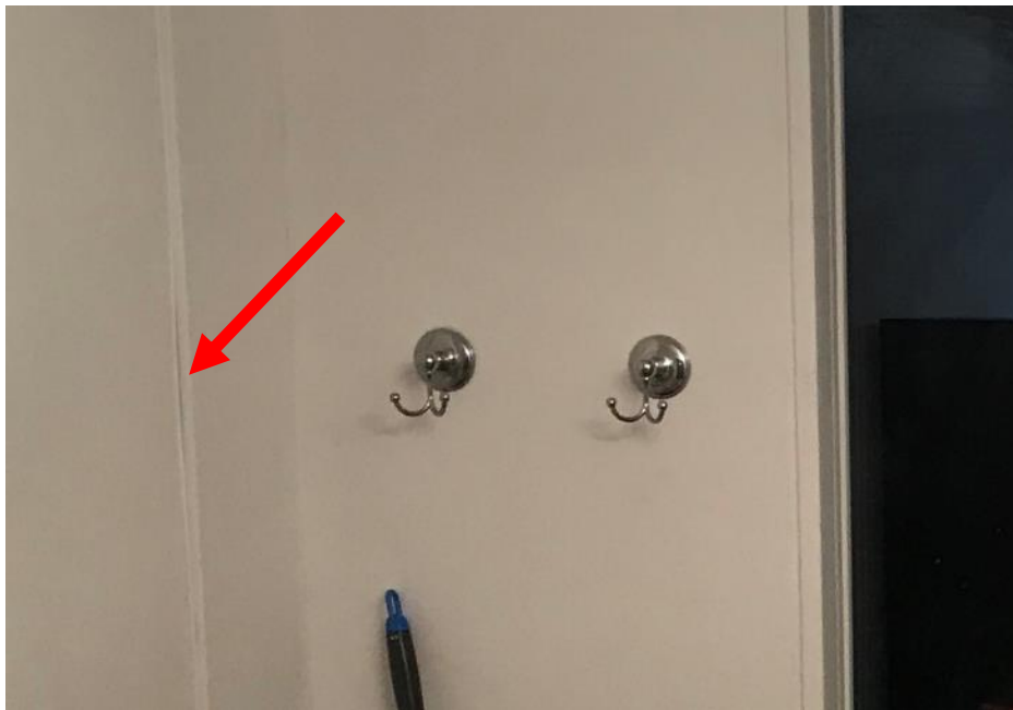
HA No. 44. Tan fiberglass reinforced panel with mastic (M)
