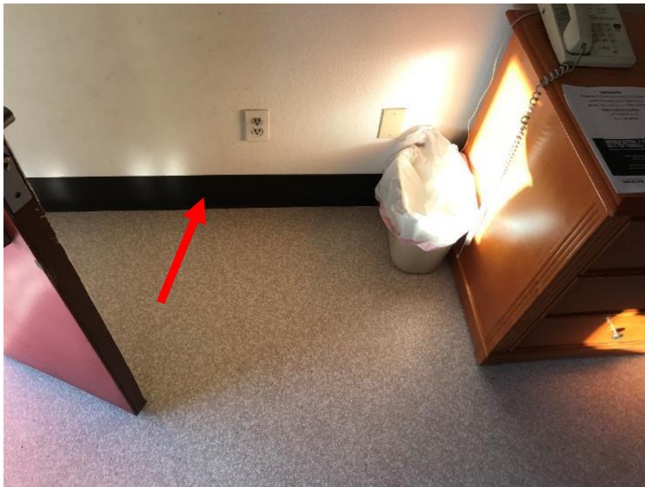
HA No. 3. 6" Brown rubber cove base, yellow mastic, and white joint compound (M)
