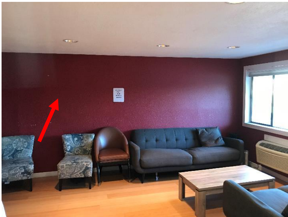
HA No. 20. White texture with mastic, white texture (S), beige wallpaper, and white joint compound (M)
