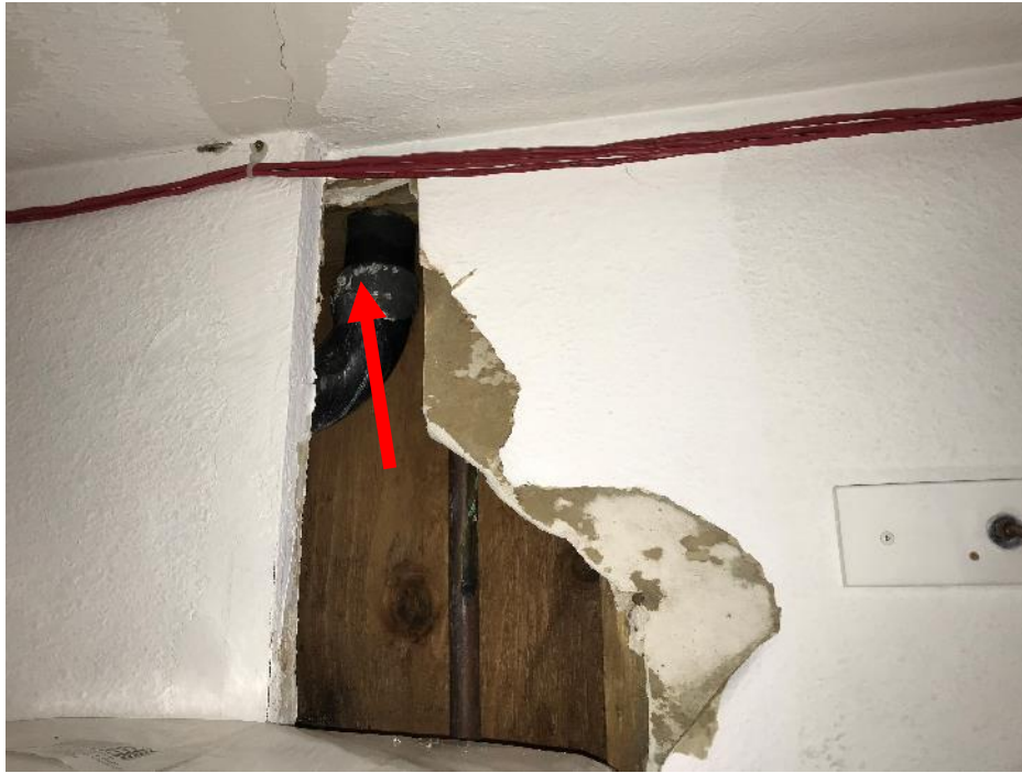
HA No. 19. Grey joint sealant (M)
