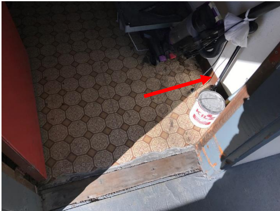
HA No. 7. 4" brown rubber cove base and beige mastic (M)
