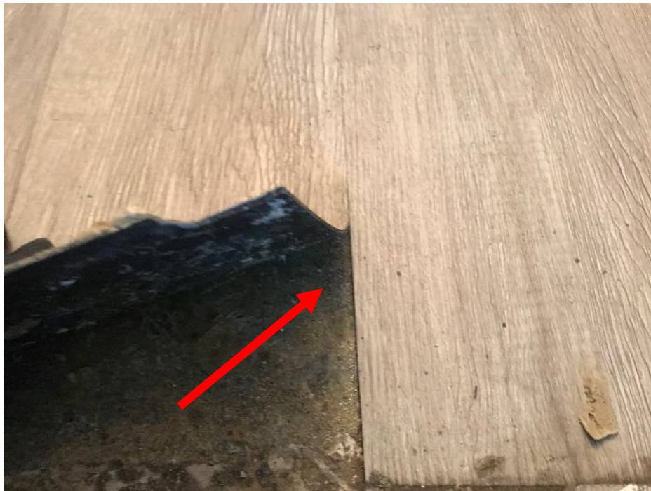
HA No. 34. Grey wood pattern vinyl floor tile, clear mastic, and grey mastic (M)
