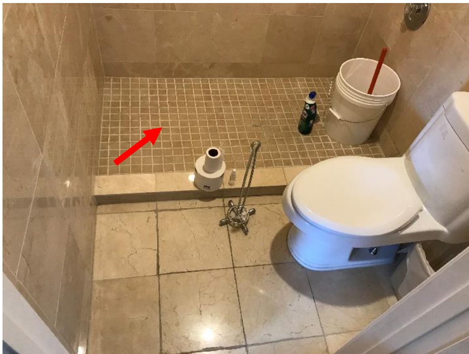
HA No. 22. 2'x 2' white and red ceramic tile, white mastic, and white grout (M)
