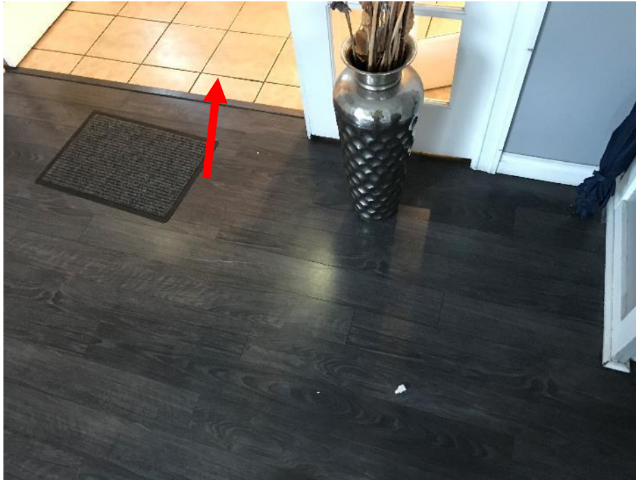
HA No. 39. 12"x 12" tan mottled ceramic floor tile, grey grout, grey mortar, and grey fibrous mat (M)
