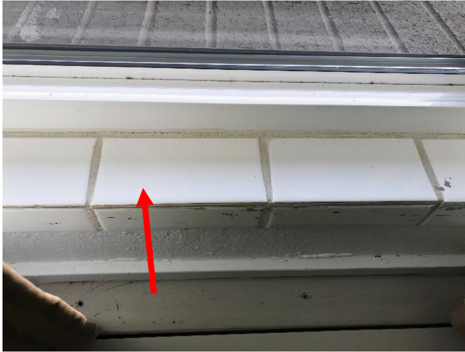
HA No. 31. 3"x 6" white ceramic tile, white grout and white material (M)
