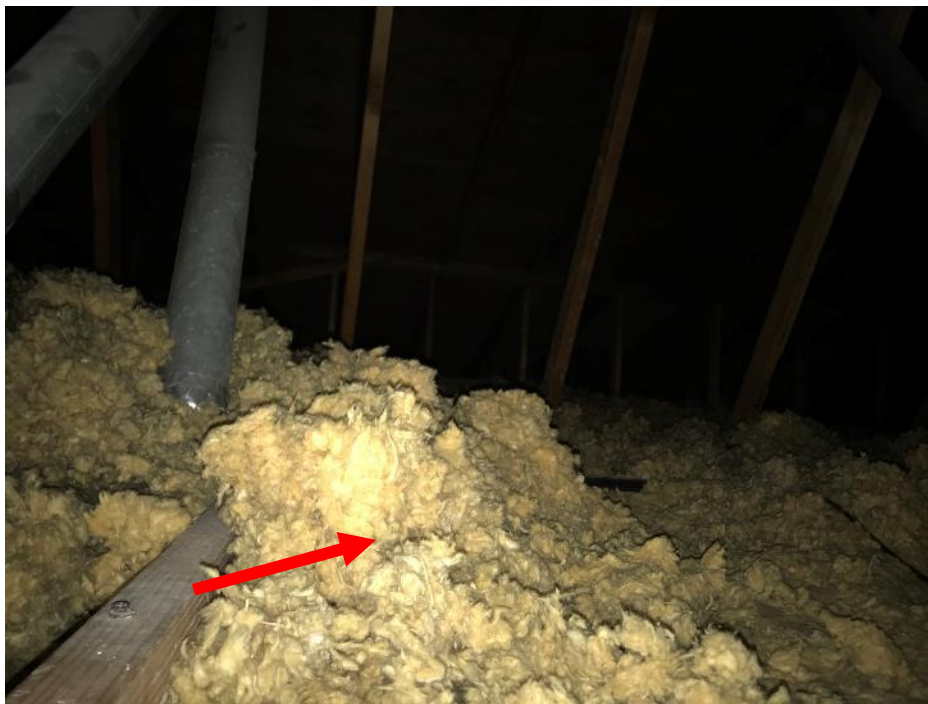
HA No. 26. Yellow fiberglass blown in insulation (T)
