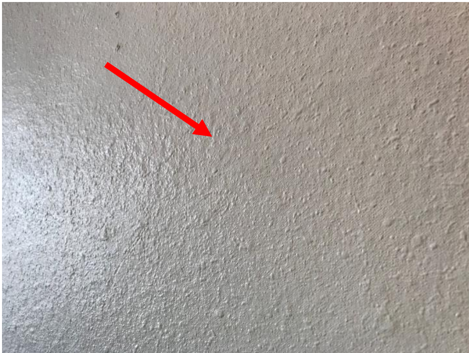
HA No. 5. White texture (S), beige wallpaper, beige mastic, white paper, and joint compound (M)
