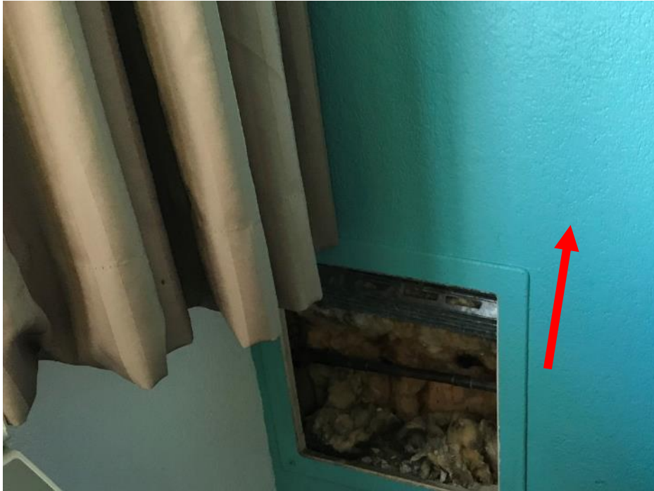
HA No. 4. White texture (S), beige wallpaper, beige mastic, white joint compound, white paper, white joint compound, white gypsum wallboard (M)
