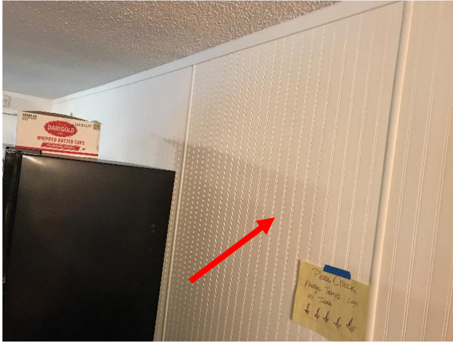
HA No. 45. Wall panel mastic (M)
