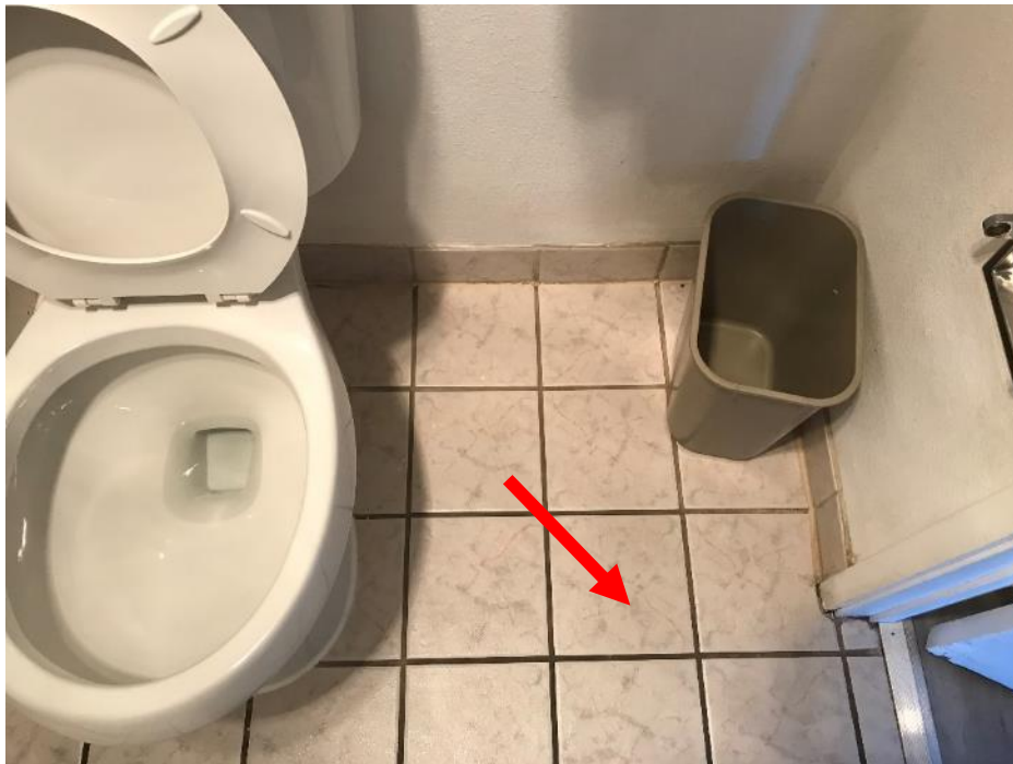
HA No. 9. 8"x 8" white ceramic tile, red grout, and grey mortar bed (M)
