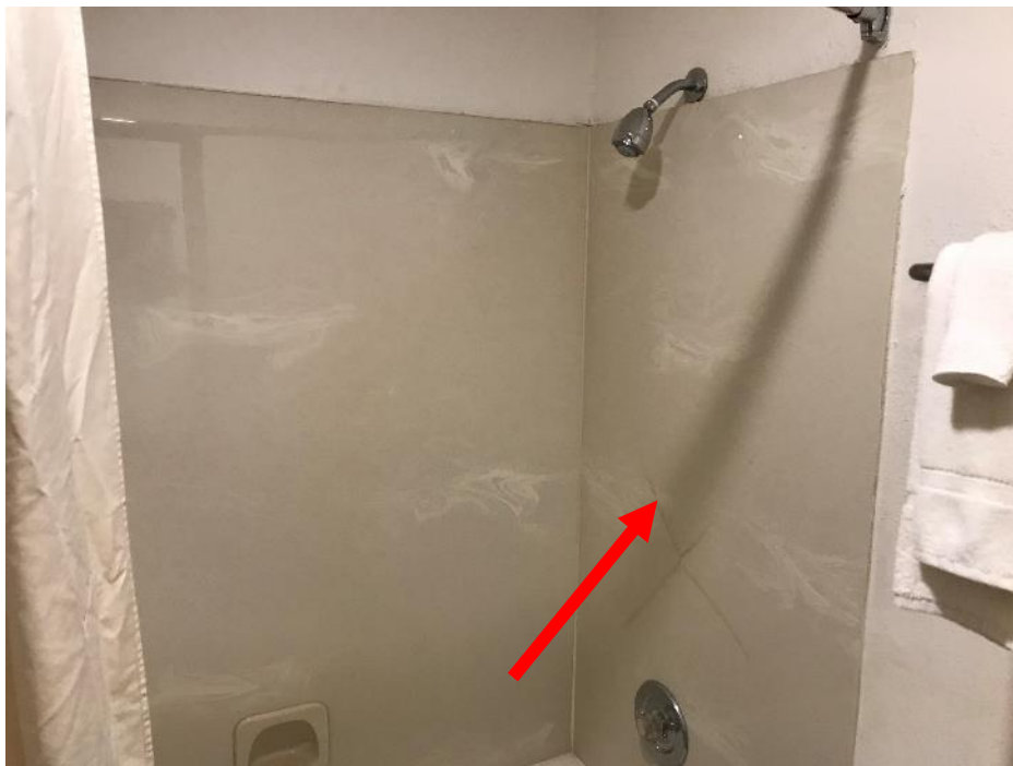
HA No. 32. Marble panel with tan grout (M)
