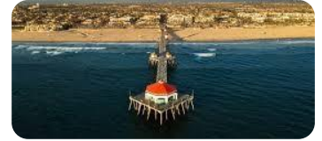
Huntington Beach Pier
